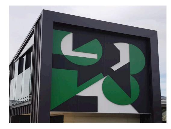
Before cutting the four powdered, coated aluminium panels, Cutshop<sup>®</sup> created a wooden template, liaising with Evonne's builder to figure out where best to place the fixings. Cutshop<sup>®</sup> also sourced a sign writer that could wrap each of the panels in green or black matt vinyl to create the pattern.
