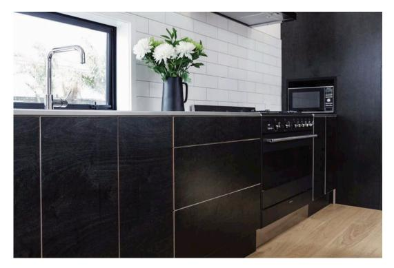
Courtney chose a prefinished 19mm PlyPlay plywood for thick, stable doors and drawer fronts. The board was UV-coated in PlyPlay's Penrose factory, and then sent to the Cutshop<sup>®</sup> to get it digitally cut for the exact drawer and cupboard sizes.
